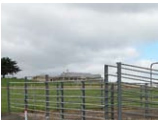
Figure 11: Well constructed yards with road access
