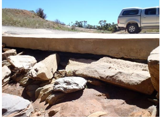
Undermining at the downstream end of a concrete ford crossing
