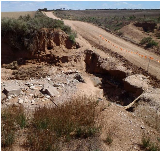
Ford crossing impacted by a downstream erosion head
