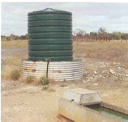
Existing trough and tank setup. The tank is elevated 1m using an old galvanised tank filled with soil.
