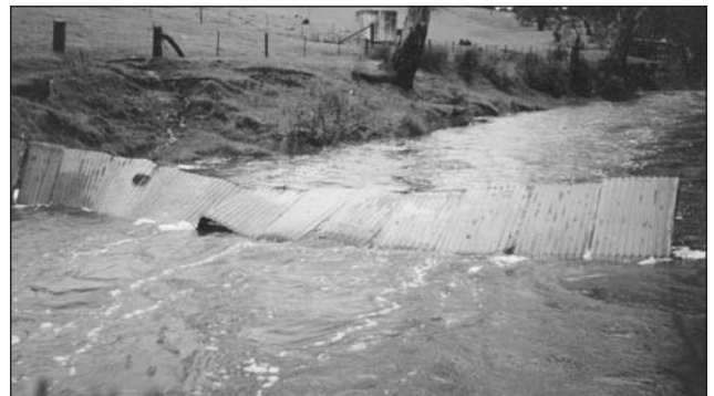
Corrugated iron floodgate... an oldie, but not necessarily a goldie
